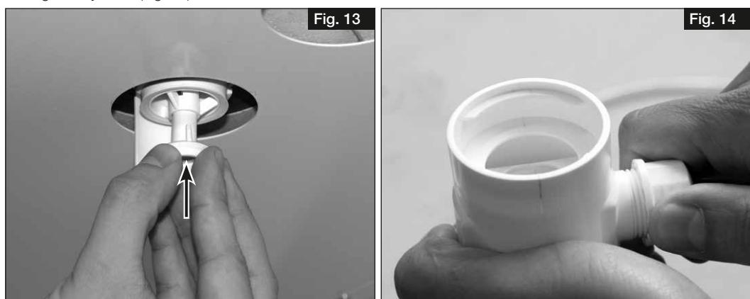
5. Connect siphon casing and turn a 1/4 turn in the mounting part (see Fig. 15). Ensure that the float ball is loose in the casing!
